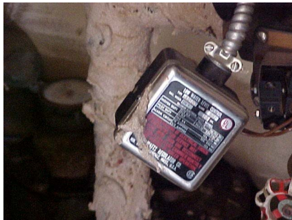
Figure 3. Low water switch box cover hanging from bracket
