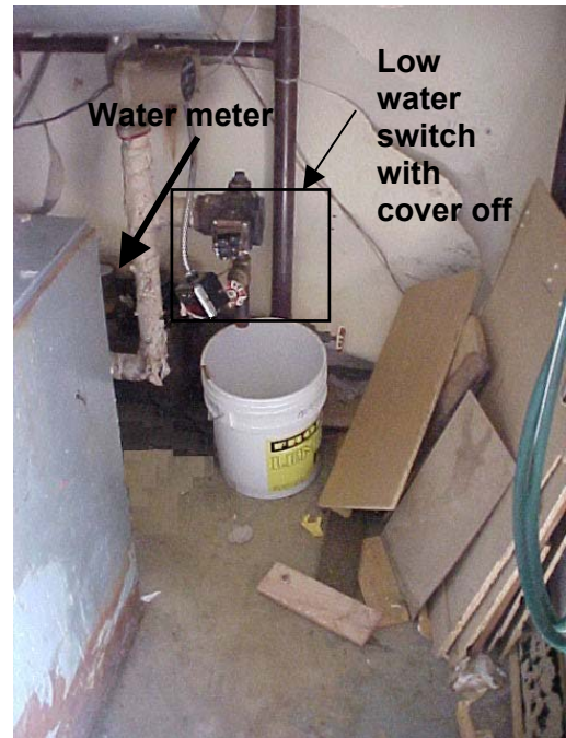
Figure 1. View of area near boiler
