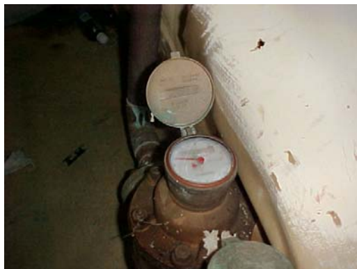
Figure 2. Water meter at floor level
