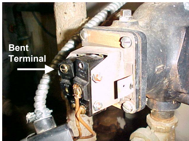
Figure 4. Low water switch terminals after victim contact
